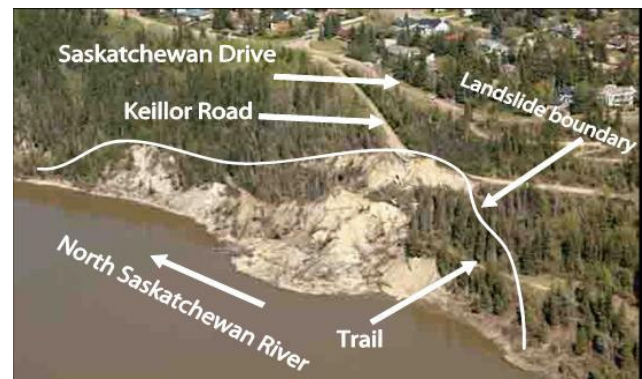
Figure 1 Keillor Road landslide (May 2005, the City of Edmonton)
